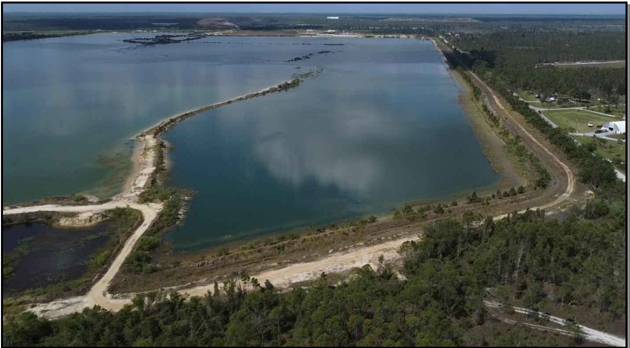
Looking west across northern portion of primary excavation pit
