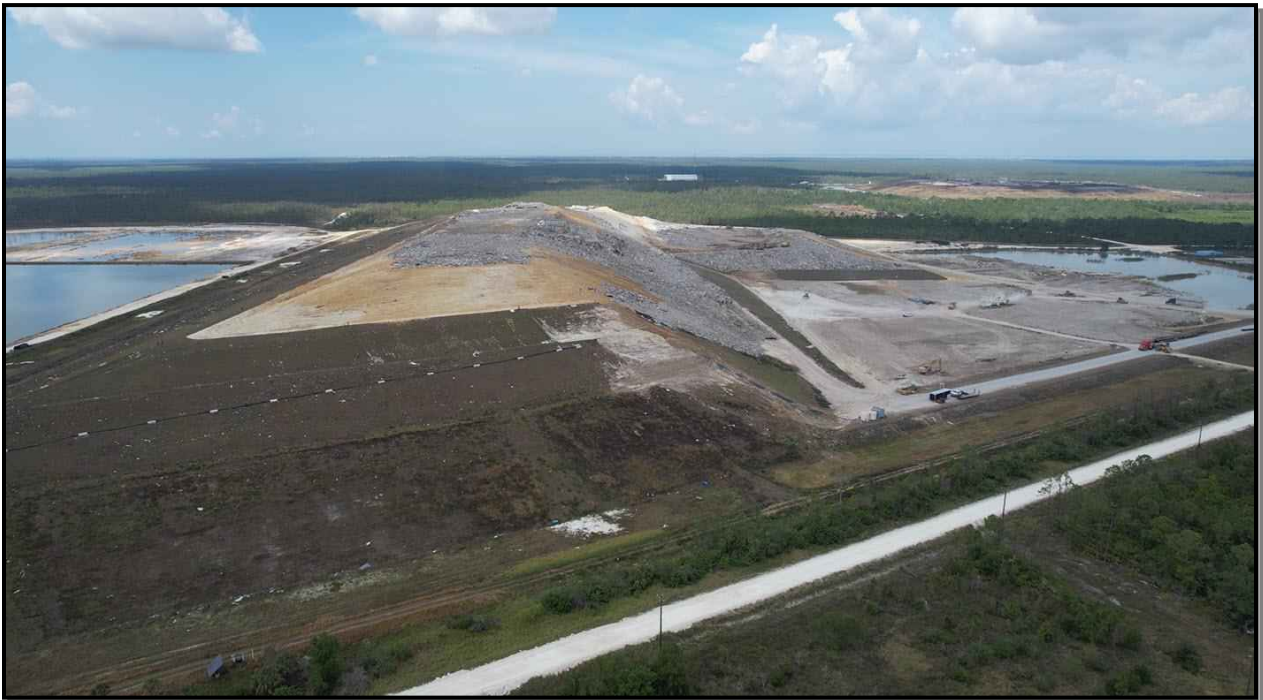
County land fill located across US 41 from the subject
