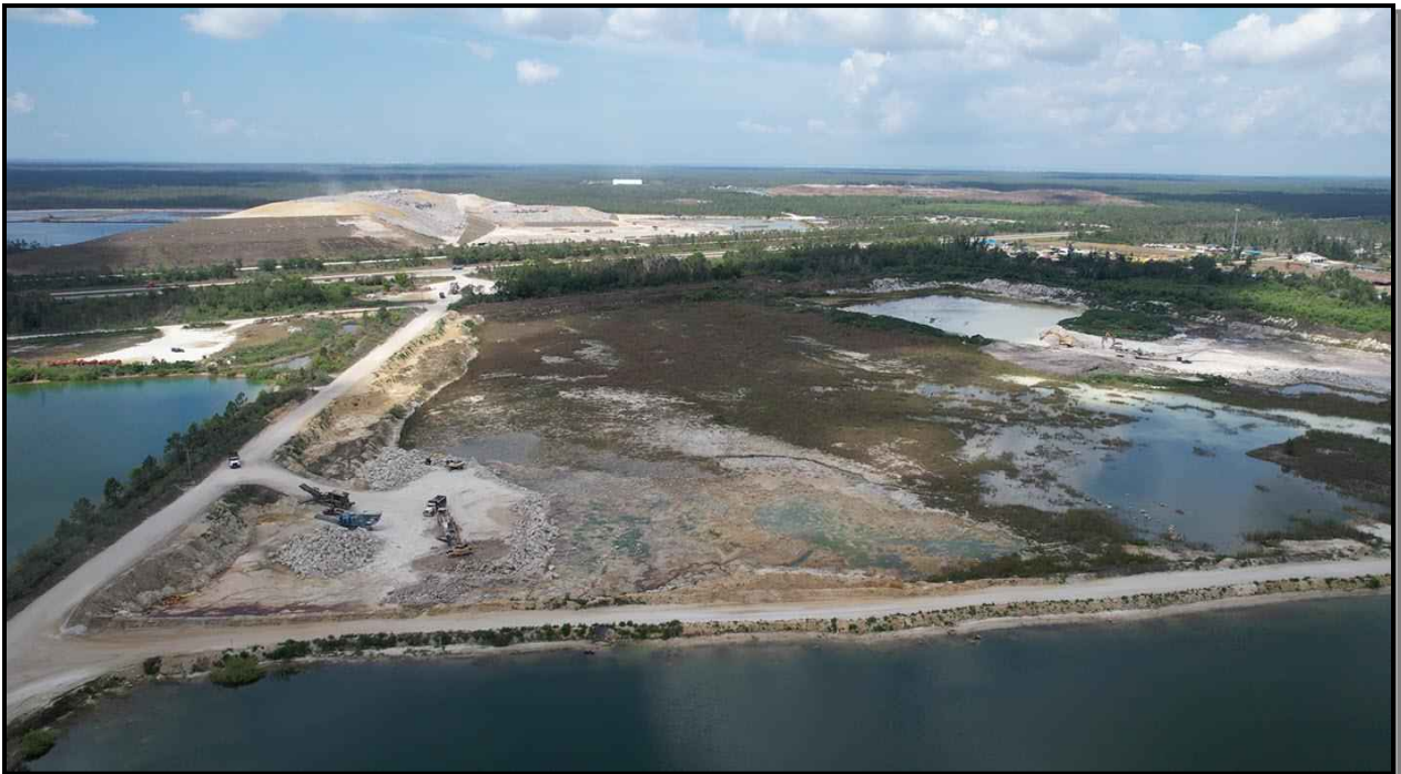
Looking west at the current excavation cell in the northwest corner of the property
